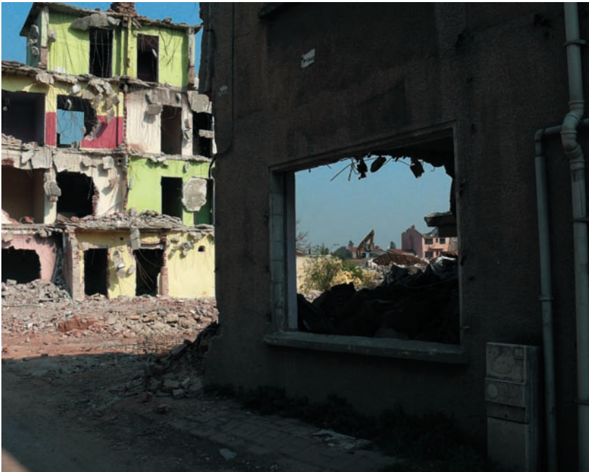
Demolition of Sulukule – Turkey.
